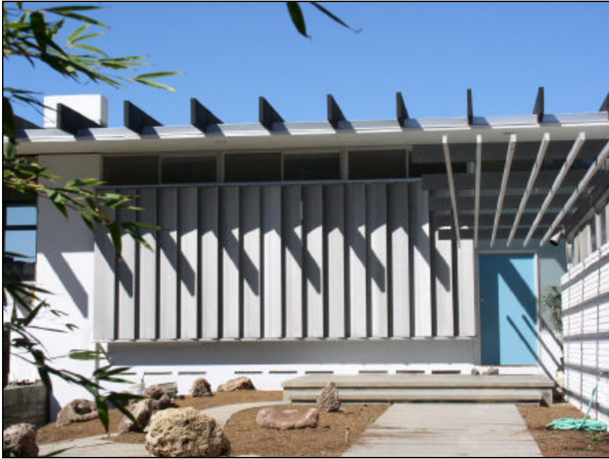
Primary (south) elevation, living room louvers closed, looking north
