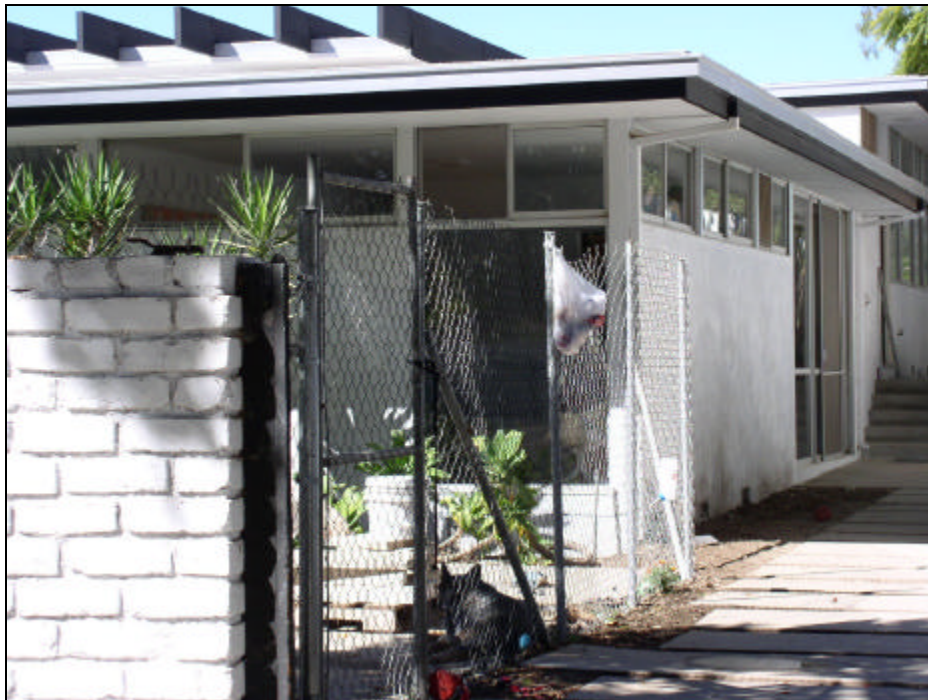
Southeast corner of residence, bedrooms and courtyard, looking northwest
