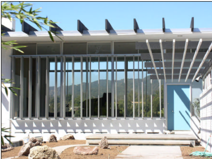
Primary (south) elevation, living room louvers open, looking north
