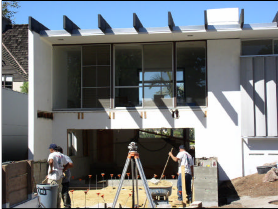
Southwest corner of residence, garage with study above, looking north
