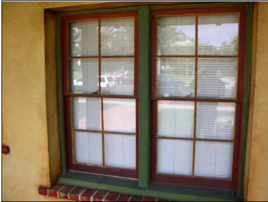
Window detail, primary (north) elevation, looking southeast
