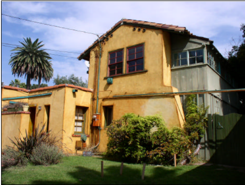
Two-story addition at south end (rear) of residence, looking northeast
