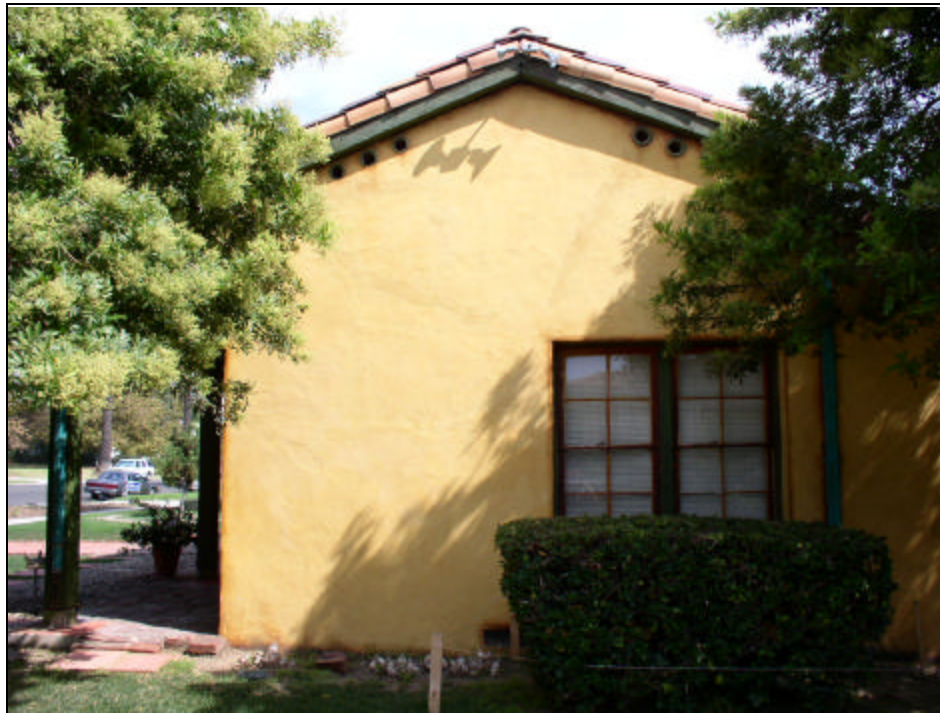
West elevation, looking east
