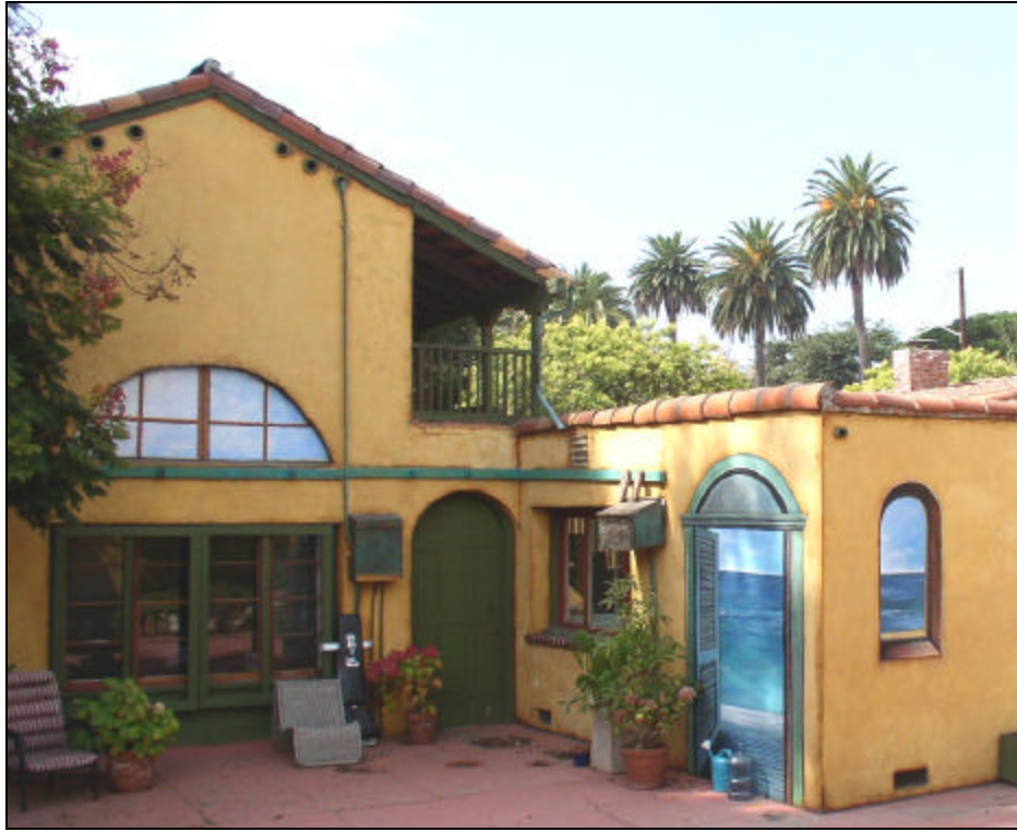
East elevation of two-story addition, looking northwest
