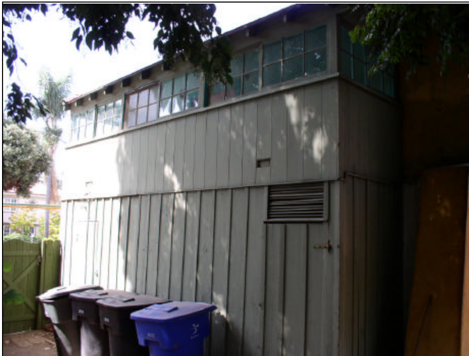
South (rear) elevation of two-story addition, looking northwest
