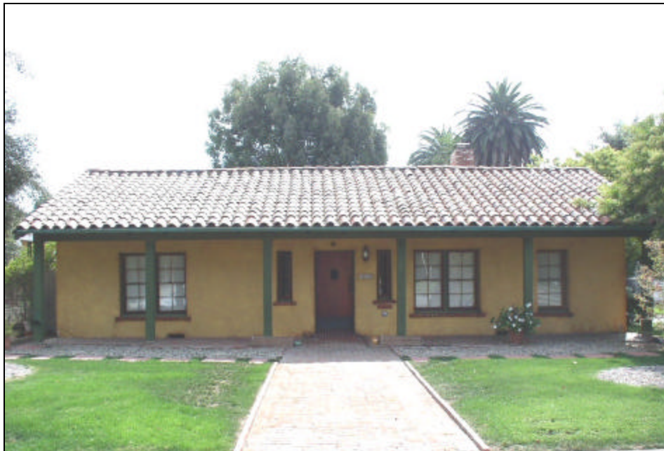
Primary (north) elevation, looking south
