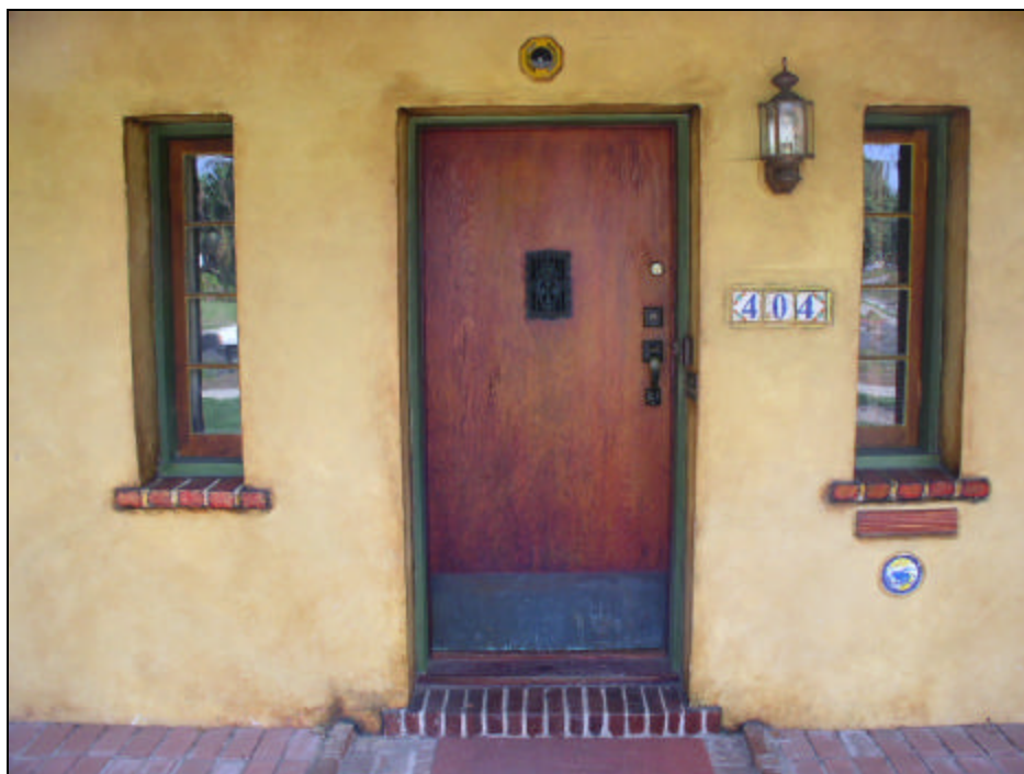
Entry detail, primary (north) elevation, looking south
