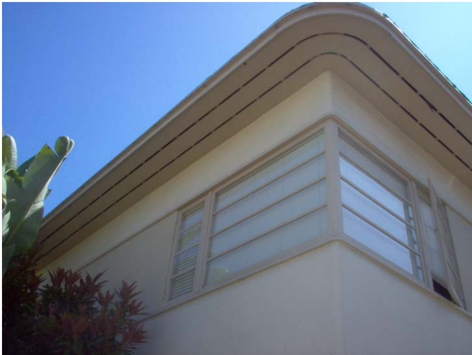
Detail, corner window and curvilinear eaves.
