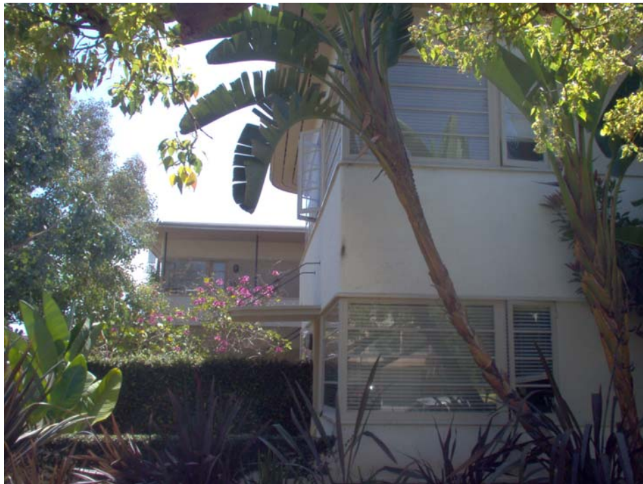
Primary (south) elevation and east elevation, view west.
