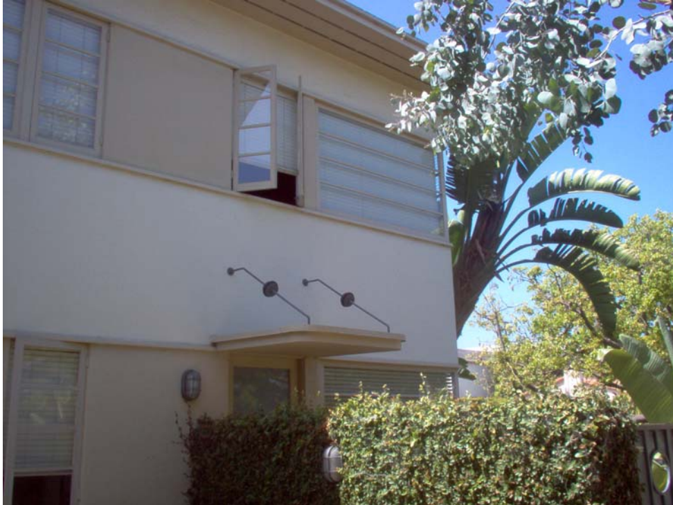
Detail, awning with metal tension cables.
