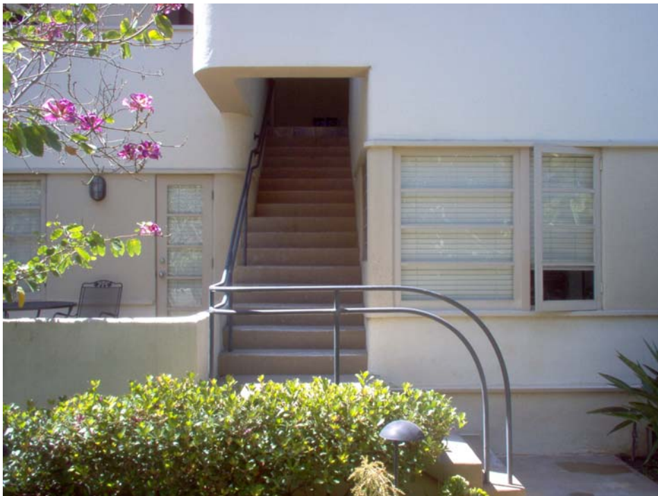
Detail, curvilinear handrail and stair.
