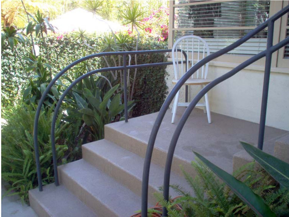
Detail, curvilinear handrails.
