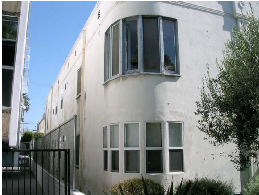
Primary (northwest corner) elevation and secondary (north) elevation, looking southeast
