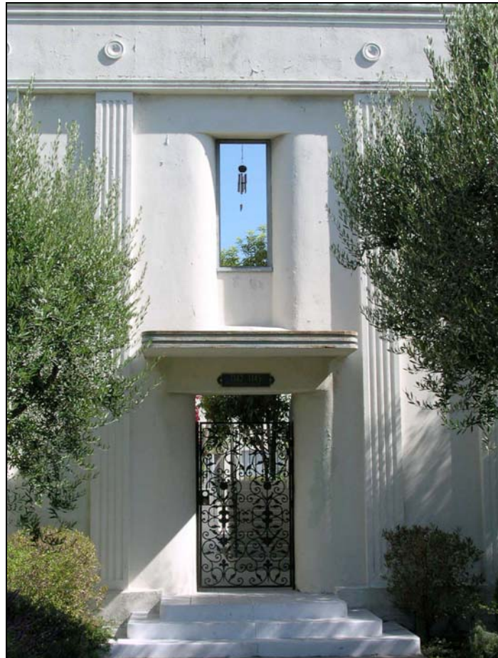
Primary (west) elevation, looking east
