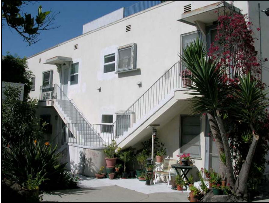
North wing, south elevation, looking northwest from paved courtyard
