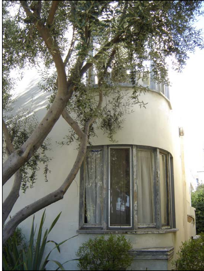
Primary (southwest corner) elevation, looking east
