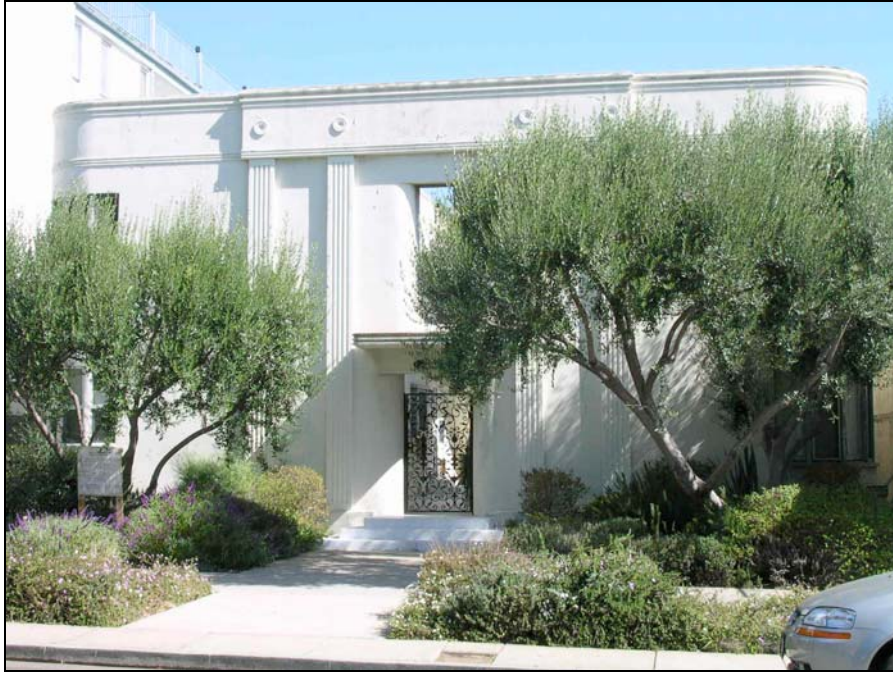
Primary (west) elevation, looking east
