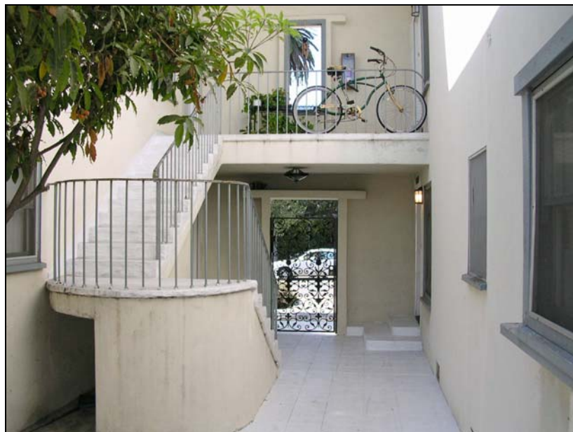
Paved interior courtyard between north and south wings, looking west
