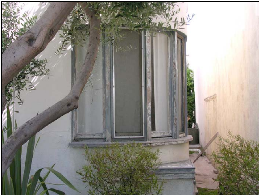
Window detail, southwest corner, looking east
