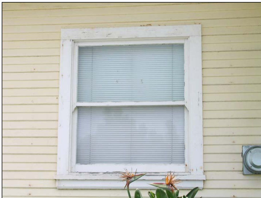
Window detail, looking east.
