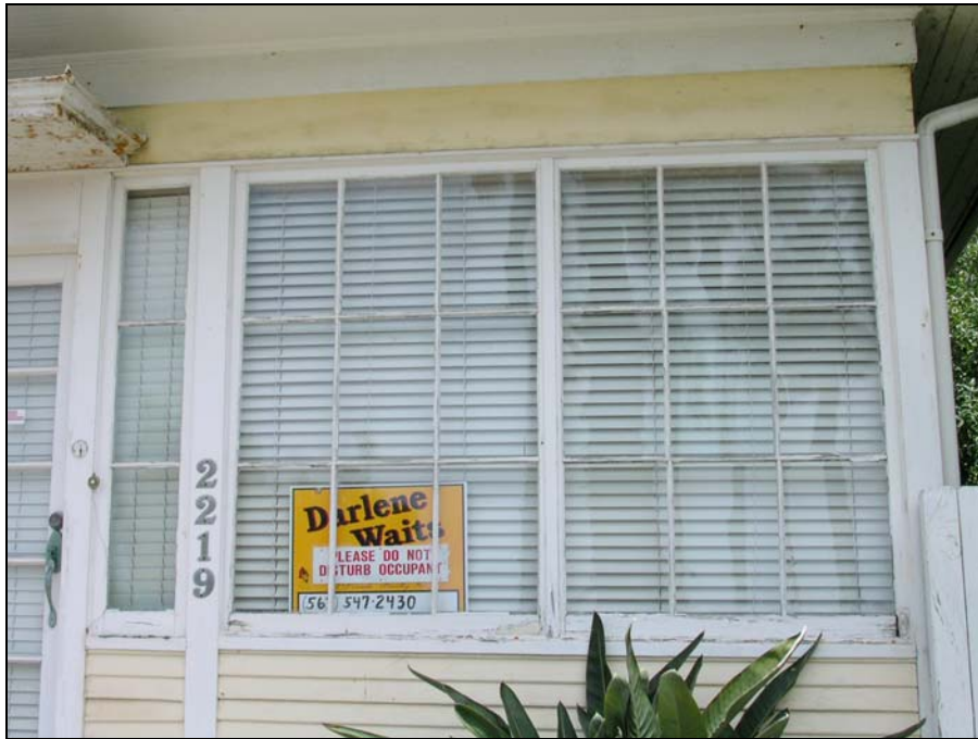
Porch fenestration detail, looking east.
