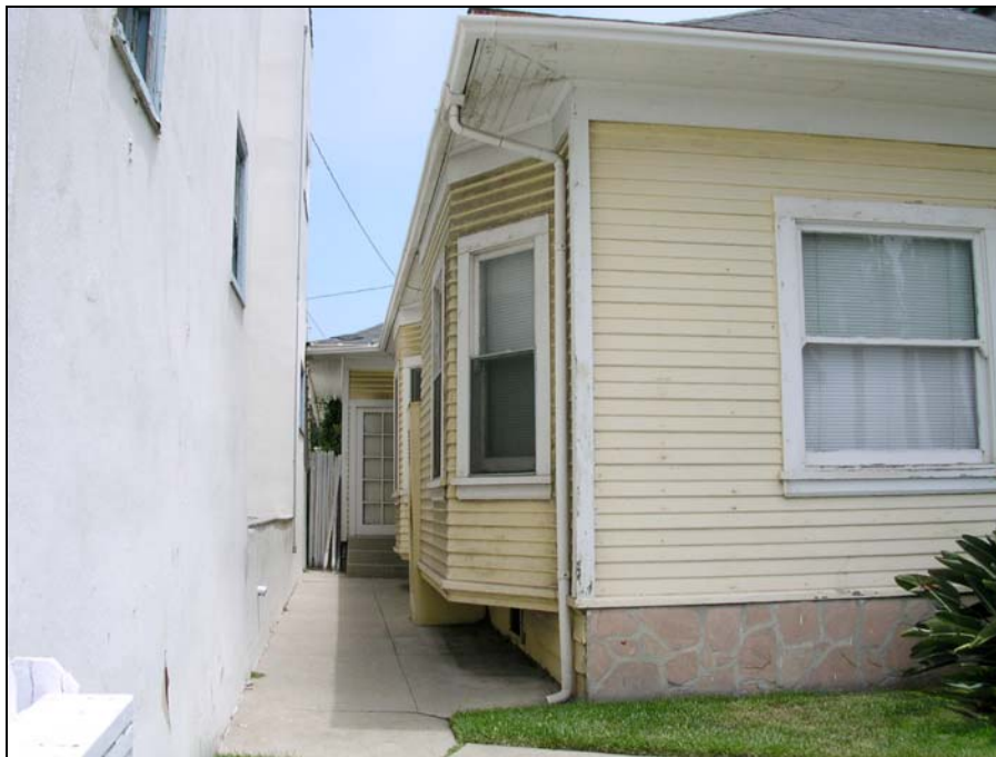
Primary (west) and secondary (north) elevations, looking east.
