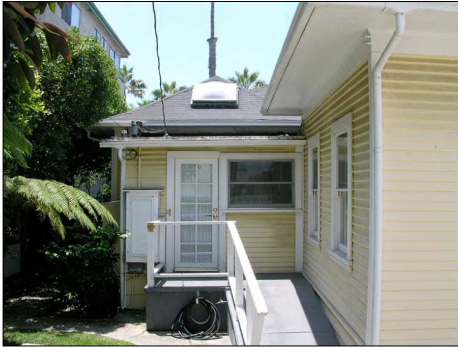
Rear (east) and south elevations, looking west.
