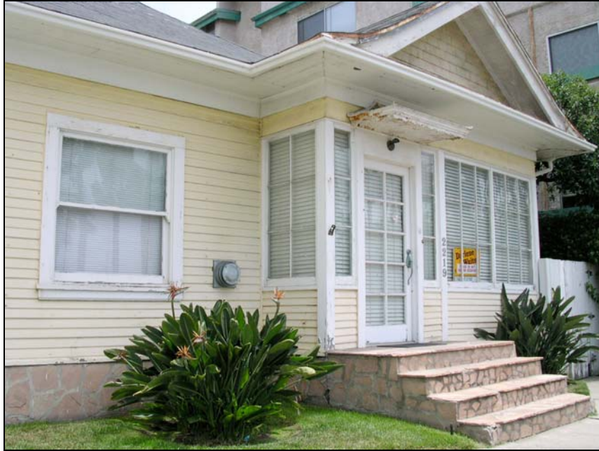
Front entry porch area, west elevation, looking southeast.
