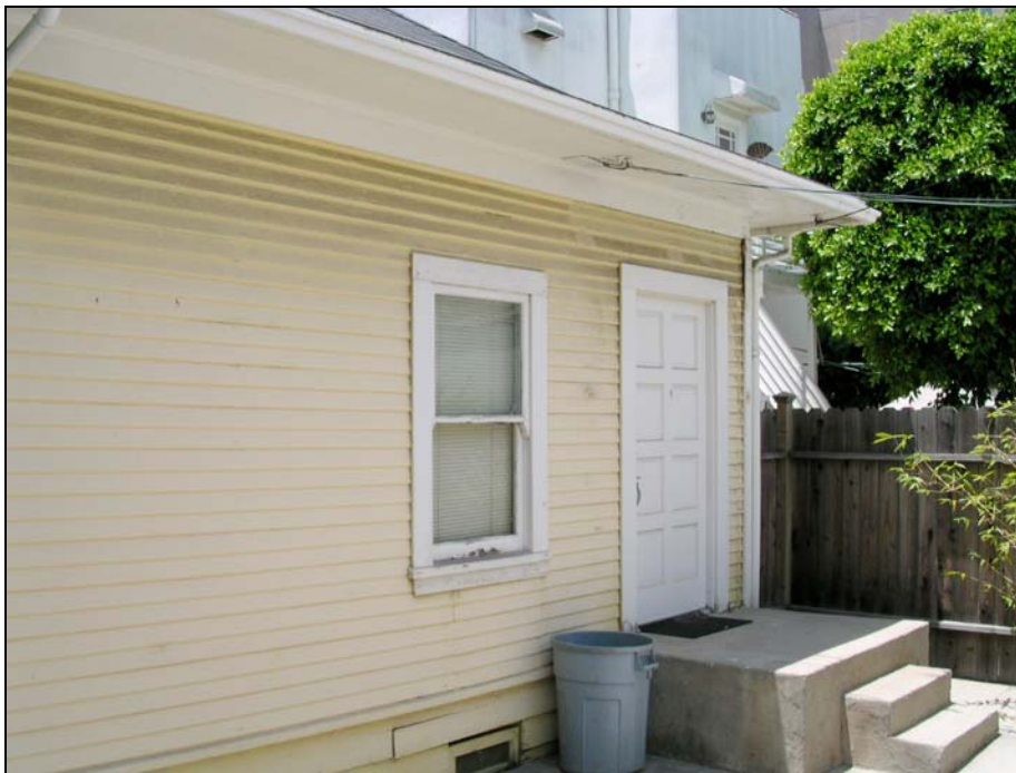
Rear (east) elevation, looking northwest.
