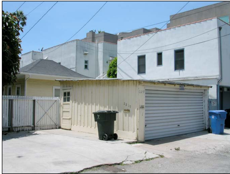
Detached rear (east) garage, looking northwest.
