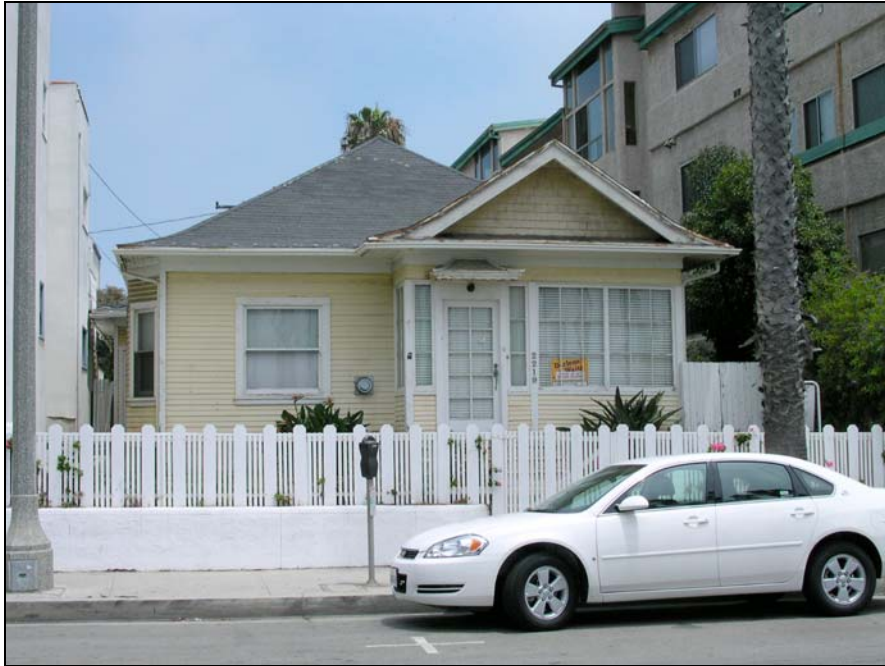
Primary (west) elevation, looking east.
