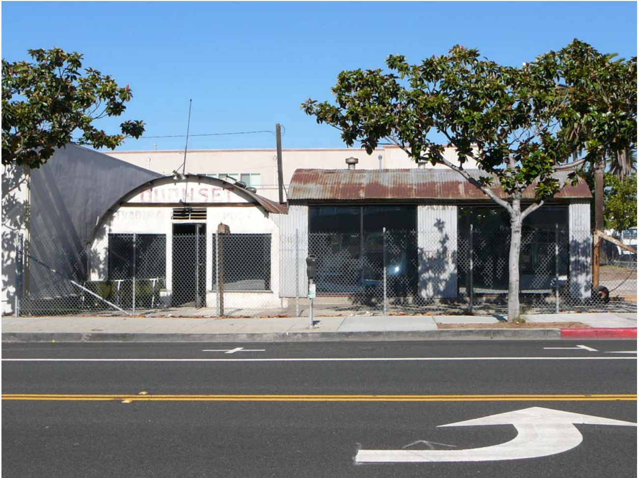
Front (South) Elevation, View North.
