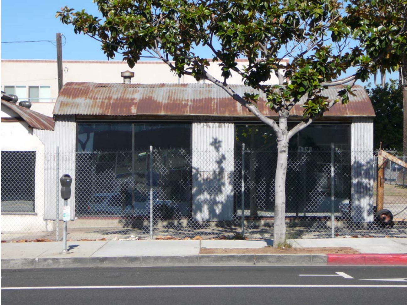
East Quonset Hut South Elevation, View North.
