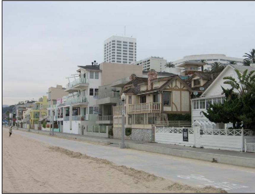
The Promenade, looking northeast. Subject property on right.
