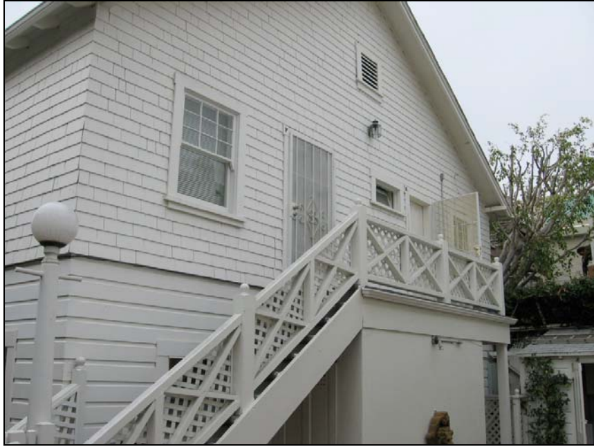
Beach-facing dwelling, rear (east) elevation, looking northwest.
