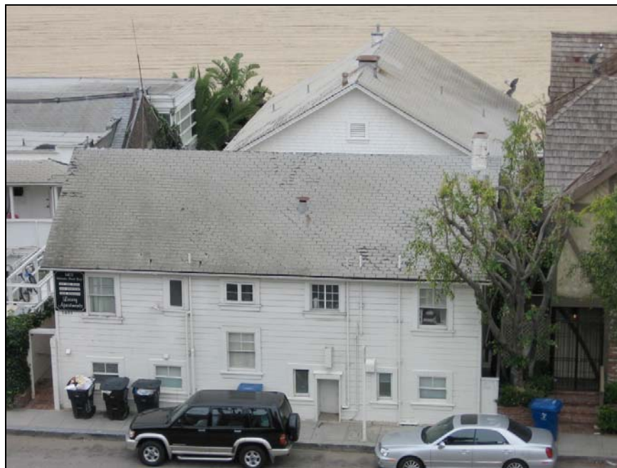
Subject property, east elevations, looking west.
