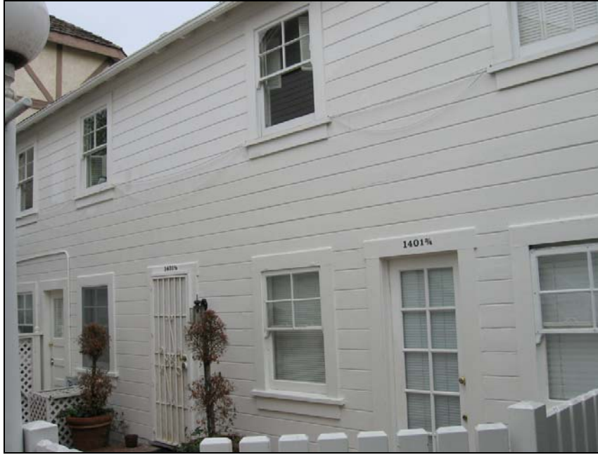
Street-facing dwelling, rear (west) elevation, looking northeast.
