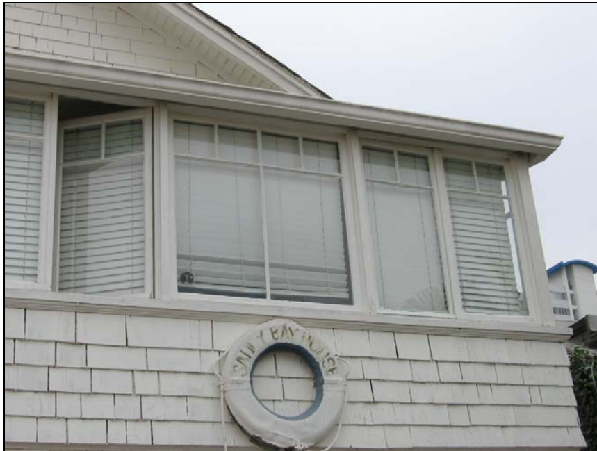
Beach-facing dwelling, window detail, looking east.
