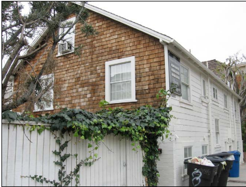
Street-facing dwelling, secondary (south) elevation, looking northwest.
