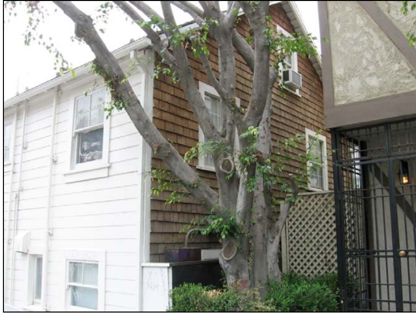
Street-facing dwelling, secondary (north) elevation, looking southwest.
