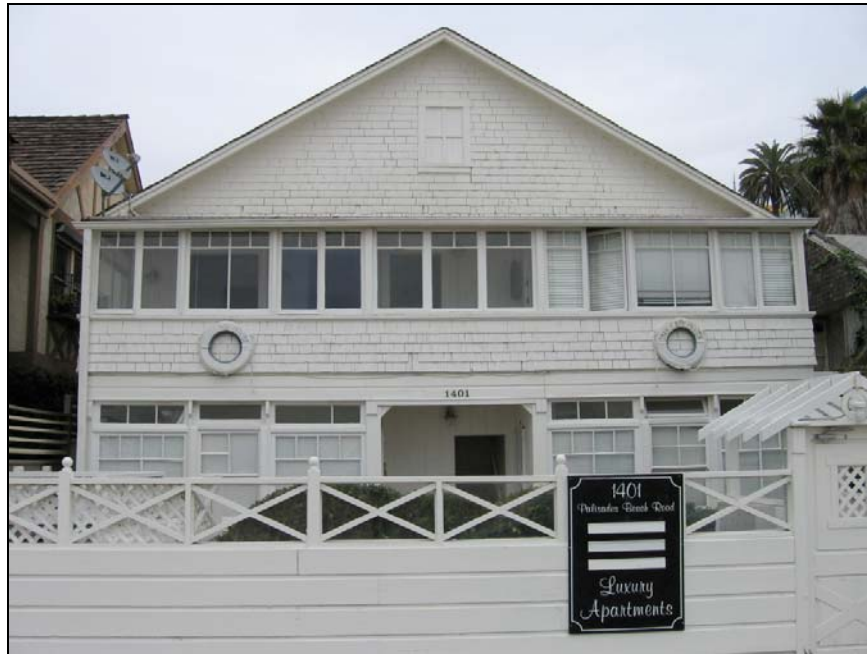
Beach-facing dwelling, primary (west) elevation, looking east.
