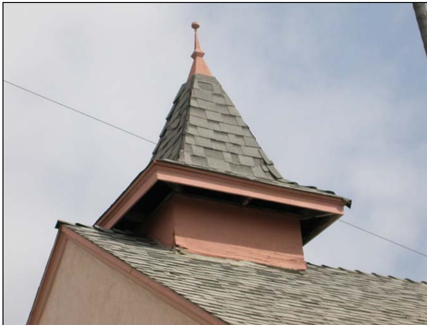
Steeple, looking northeast.
