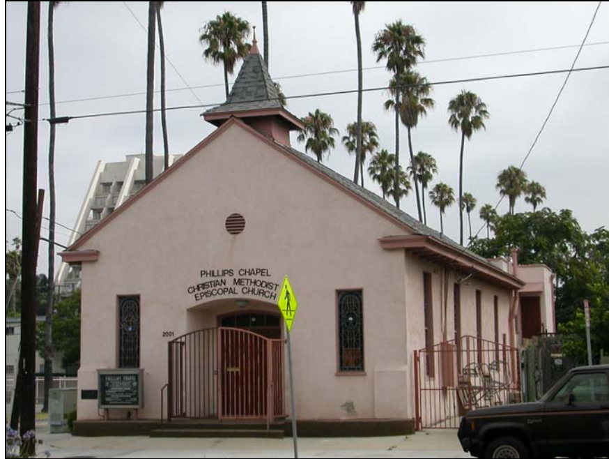
Primary (west) and south elevations, looking northeast.
