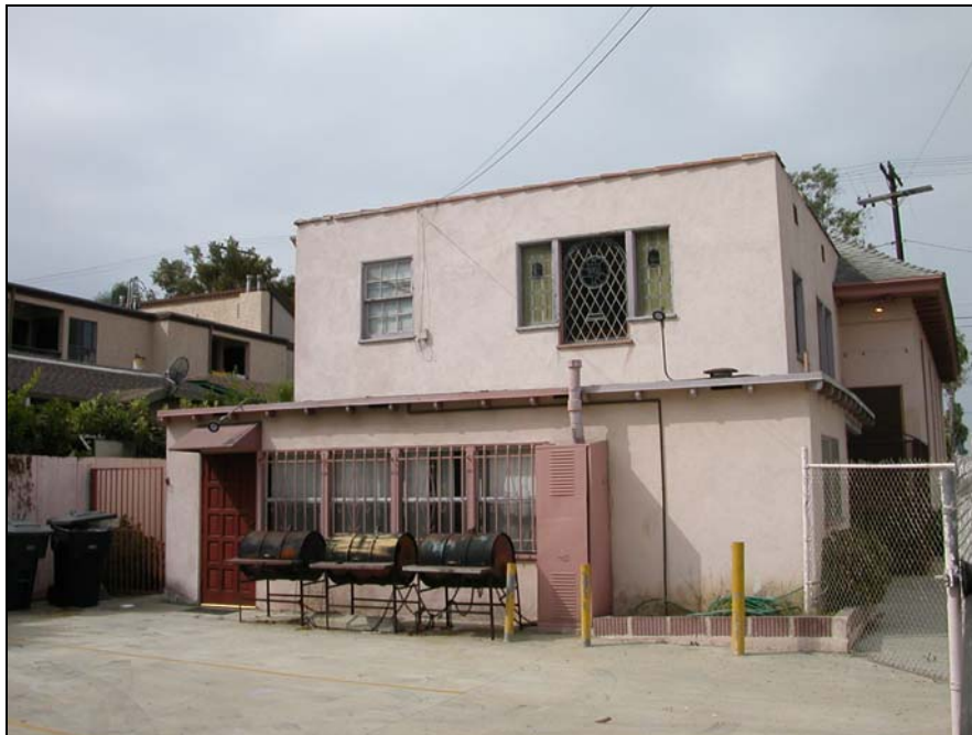
East elevation, looking southwest.
