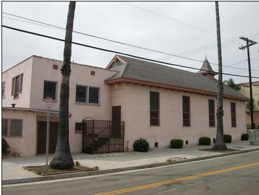
Primary (north) elevation, looking southwest.
