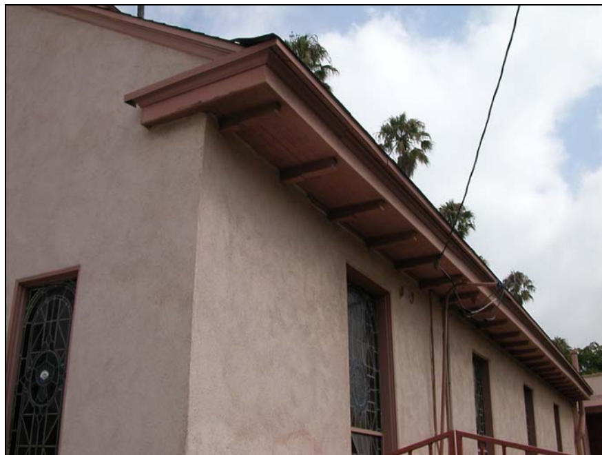
Roof detail, looking northeast.
