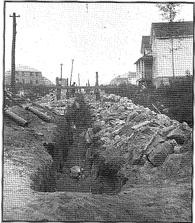
Sewer Trench on Kipawa Road, August 1919.
