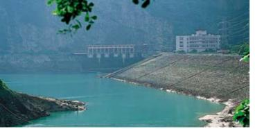
Behind the Minghu Reservoir is the Mingtan Reservoir, which was completed in 1995. It is one of the largest draw/store hydraulic power plants in the world. The Mingtan Power plant uses the Sun Moon Lake as its upper pond and the dam built in the Shuili Creek Valley as its lower pond to generate power by using the 380 meters of drop between these two ponds.
