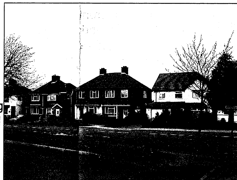
Elevations opposite proposed site indicating a mix of elevational styles
