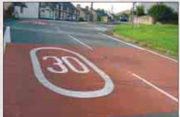
Road markings in Llanaelhaearn
