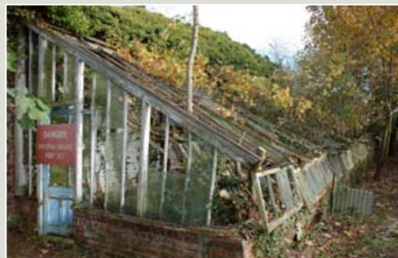
Burton Manor glasshouse before restoration
