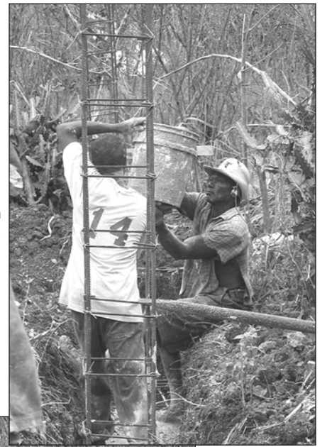
Laying the foundation by hand.
