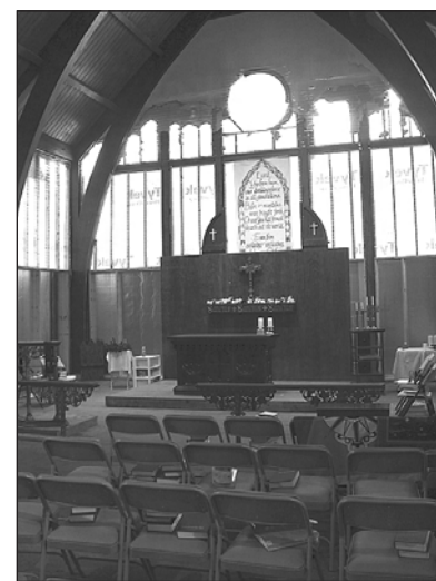
Trinity Church, in the process of rebuilding, in Pass Christian, Mississippi
