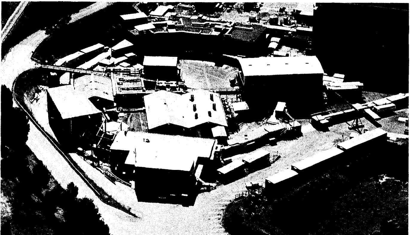
SPEAR — THE SECOND STANFORD COLLIDER The storage ring SPEAR , in the center of the photograph, was the second Stanford colliding beam machine and the first built at SLAC. The beams enter in two lines at the top right. Many of the buildings surrounding the oval ring are for experiments using synchrotron radiation, a byproduct of the stored beam.
