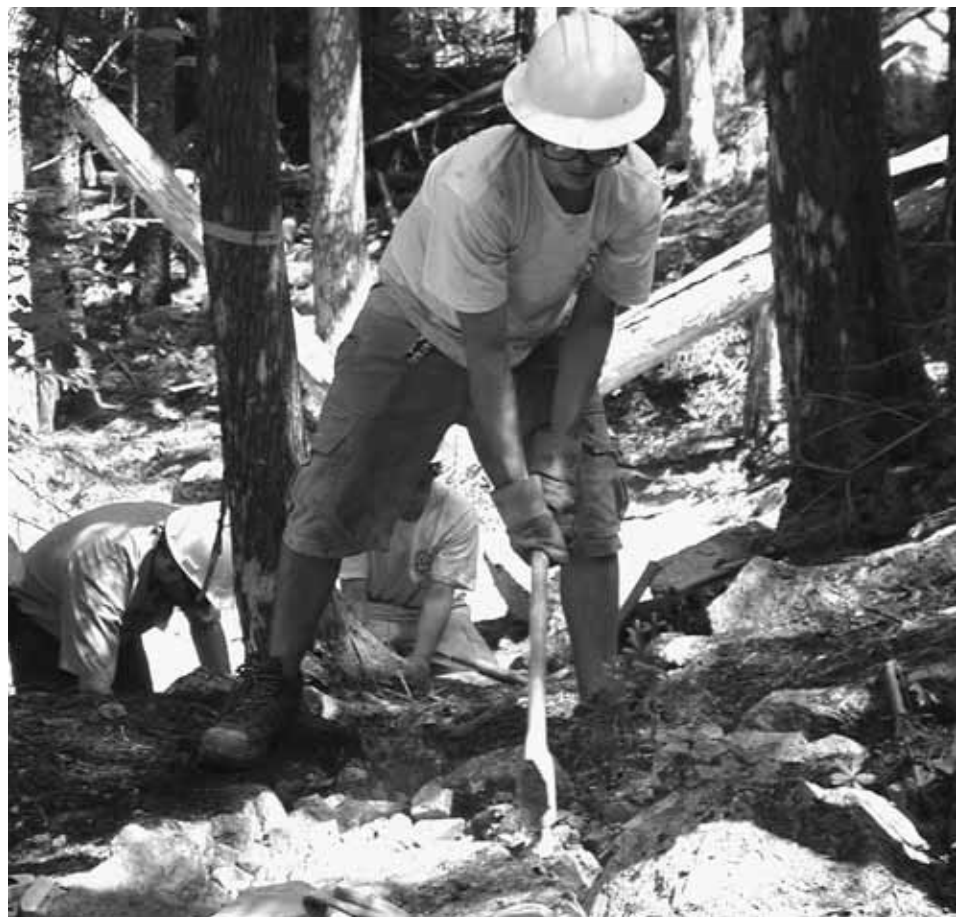
Crushing rock for trail base layer on the Maple Spring Trail.
