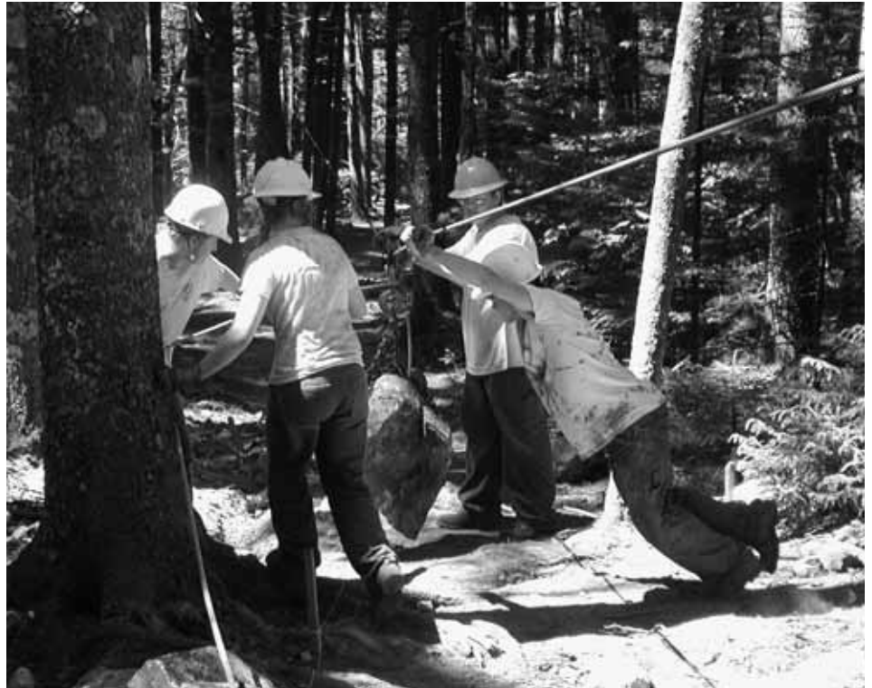
Moving rock with a high line on the Pond Trail.
