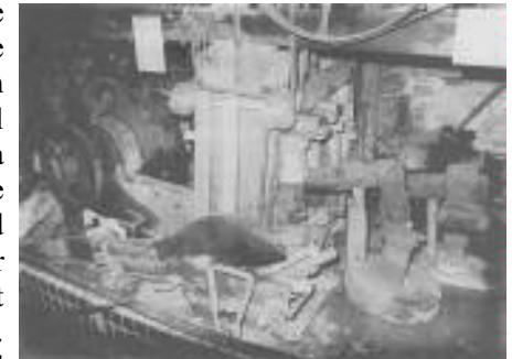
Water powered plating and steeling tilt hammers and shears at the Finch Foundry, Sticklepath
