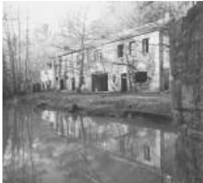
The ‘office block’ across the millpond - 1970s
