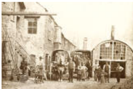
Mells Lower Works from entrance in the 1880s
