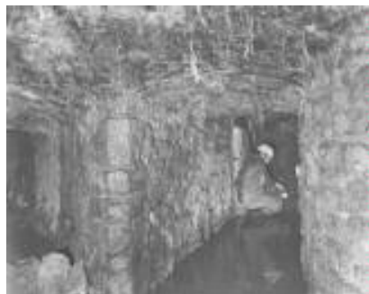
Underground water channels at Lower Works
