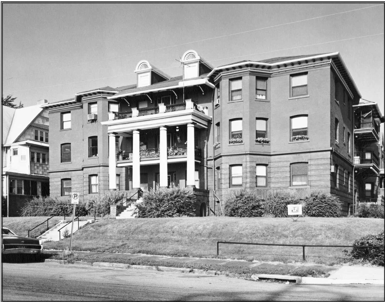
Photo 1 of 1 — looking southwest at main façade. Photo by Lynn Meyer, 1991, Omaha City Planning Department.
