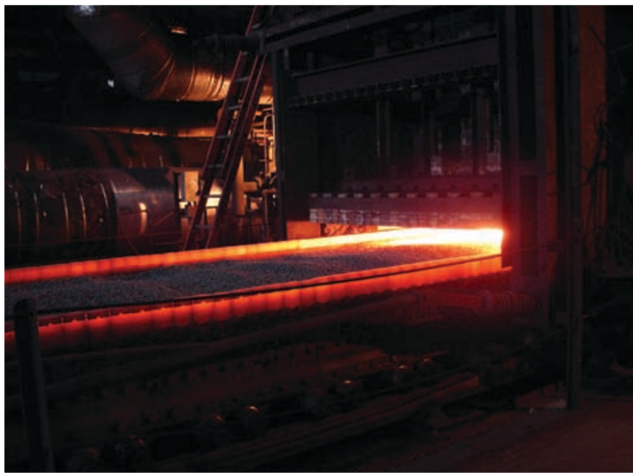
Furnace #5 at Northshore Mining Company, Silver Bay.
