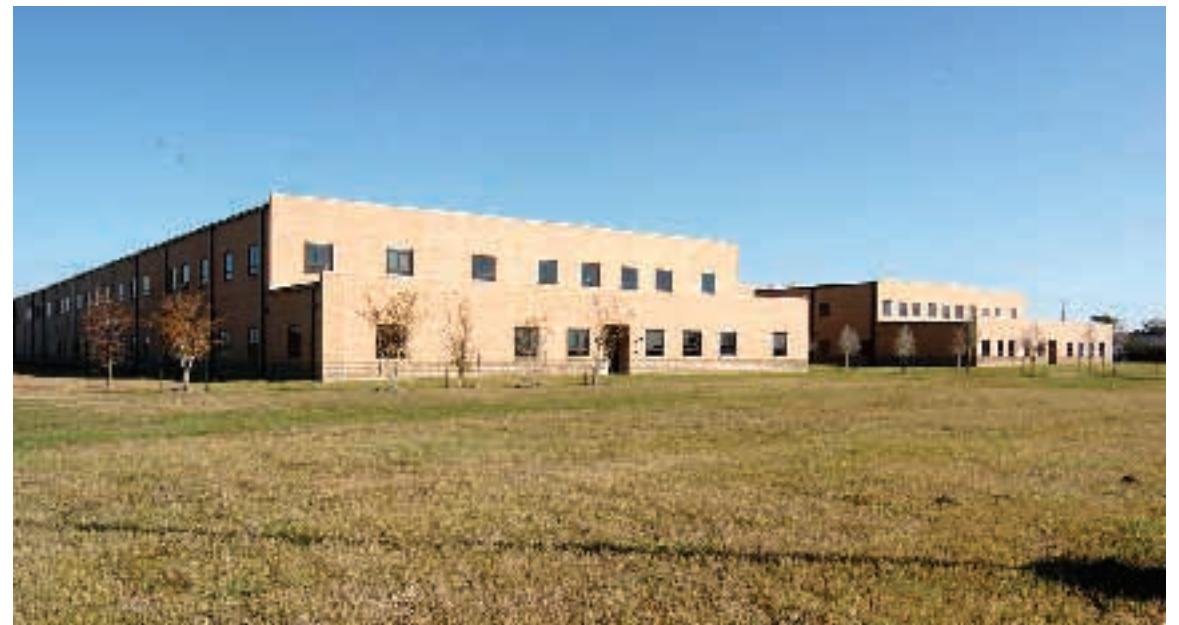
USAR occupants include the 4005th United States Army Hospital, 1st Battalion, 289th Regiment, 416th Engineer Battalion and the 10th Battalion, 95th Division, Institutional Training. Phase II scheduled for 2011, will include the construction of a 43,000 sq. ft. Battle Projection Center.
