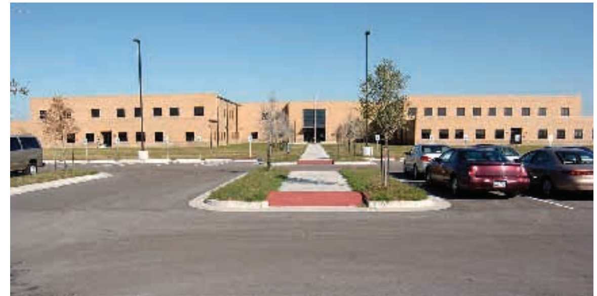
The 75th Battle Command Training Division Headquarters and 1st Brigade moved to the Armed Forces Reserve Center located at 14555 Scholl Street, Houston, Texas in November 2008. The 173,000 sq. ft., $35 million dollar facility occupies over 43 acres and serves as a Joint Reserve Center located at Ellington Field. Marine Corps and Naval Reserve units will also occupy offices within the facility.
