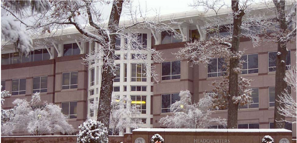
A winter scene at the headquarters building, US Army Reserve Command, Fort McPherson, Georgia, 19 December 2000. (Photo by Susan Norvick, Multi-media Specialist, Training Support Center, Fort McPherson, Georgia.)
