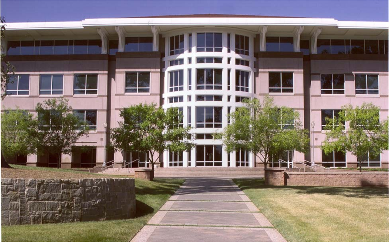
The headquarters building, US Army Reserve Command (USARC), located at Fort McPherson, Georgia. The building, completed in 1997, is part-time home to the chief of the Army Reserve, who also serves as the commanding general, USARC, 26 September 2000. (Taken by Sean Quinn, Training Support Center, Fort McPherson, Georgia.)
