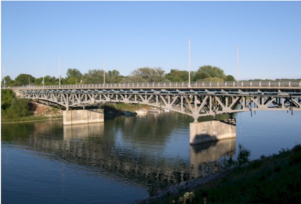
Southampton Bridge, 1959 (Saugeen River)
