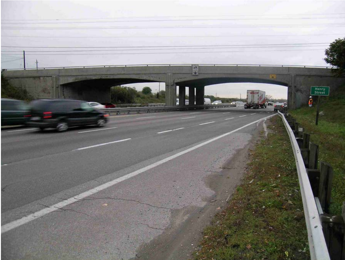
Henry Street Bridge, 1940 (Whitby)
