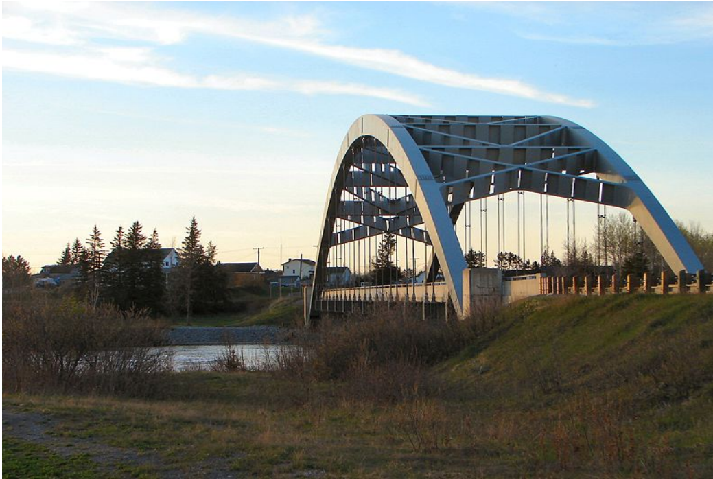
Montreal River Bridge, 1960 (Latchford)
