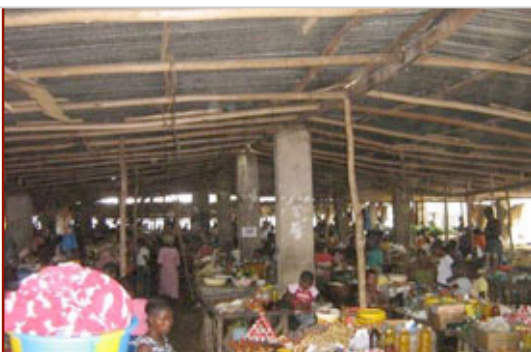
An example of an open shed
