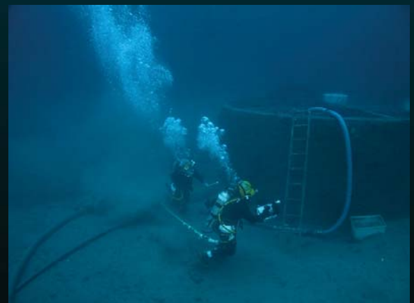
Surface supplied divers, affectionately known as sprint divers, make their way to the turret. Photo by Fleet Combat Camera, Atlantic.
