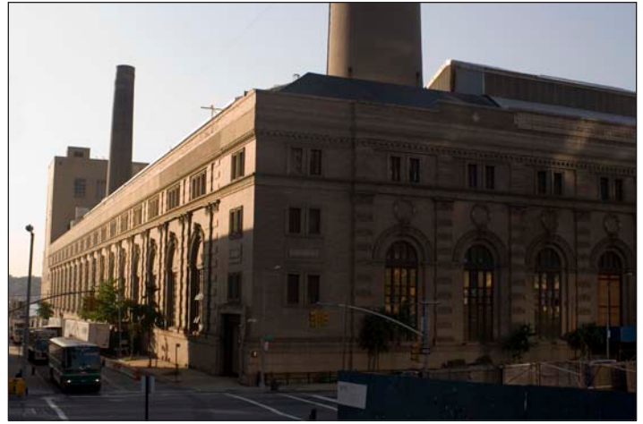
THE POWERHOUSE FILLS AN ENTIRE CITY BLOCK
