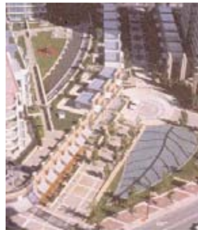
In Vancouver, townhouses surround a parking structure. Terraces and outdoor landscape space are built over the parking.
