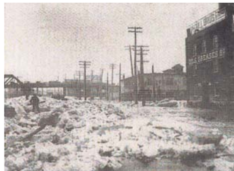
View along the rail bridge during a flood
