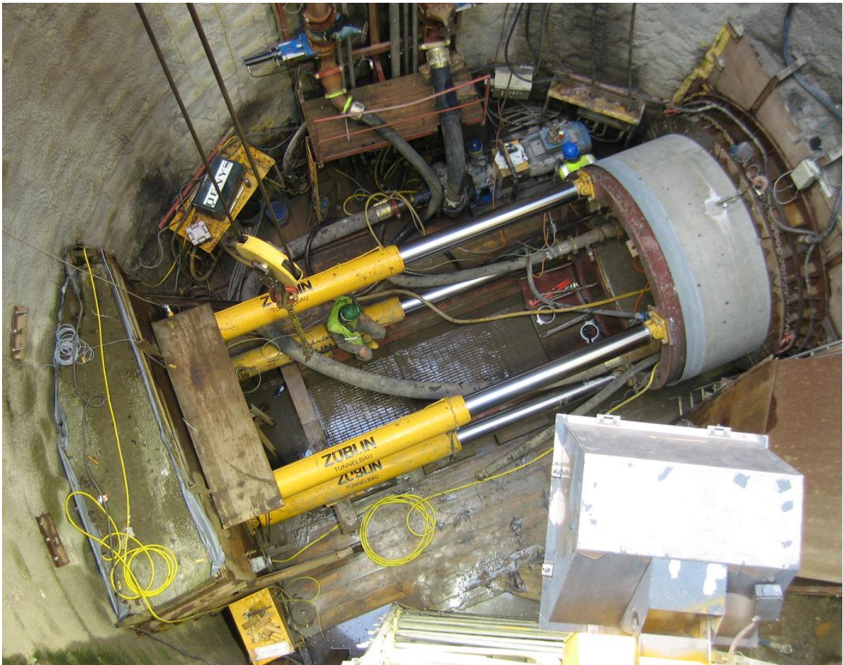
Inside the South Shaft – Jacking of Precast Concrete Tunnel Segments
