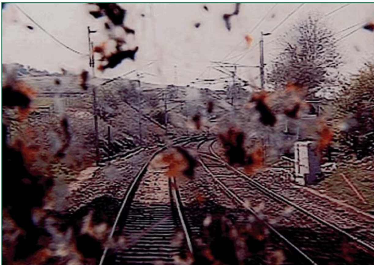
Figure 47: Approach to Lambrigg viewed from the up line in May 2006. Scrap rail behind location cabinet is visible
