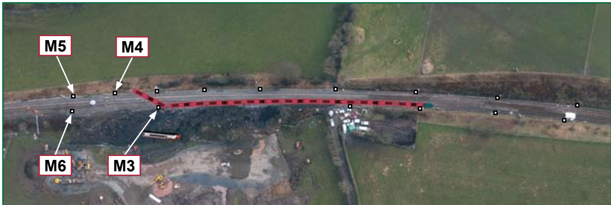
Figure 35: Reconstruction of vehicle two first striking overhead line equipment mast M3
