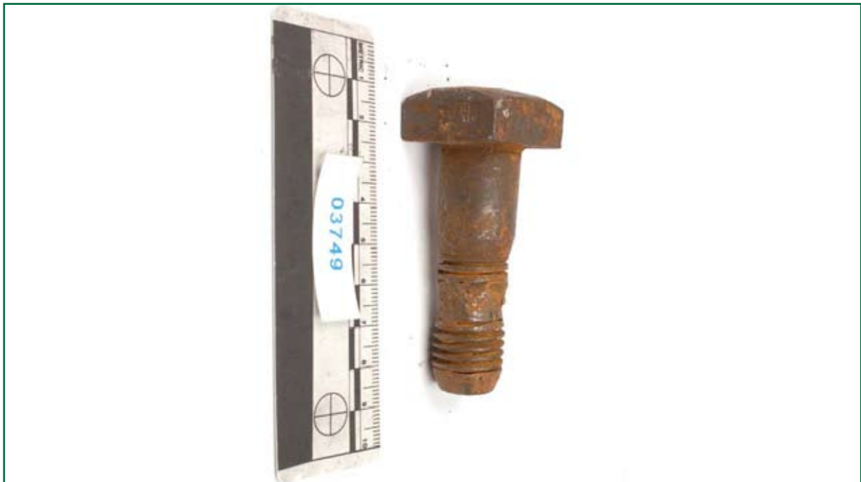
Figure 24: Damaged bolt from right-hand end bracket of third permanent way stretcher bar
