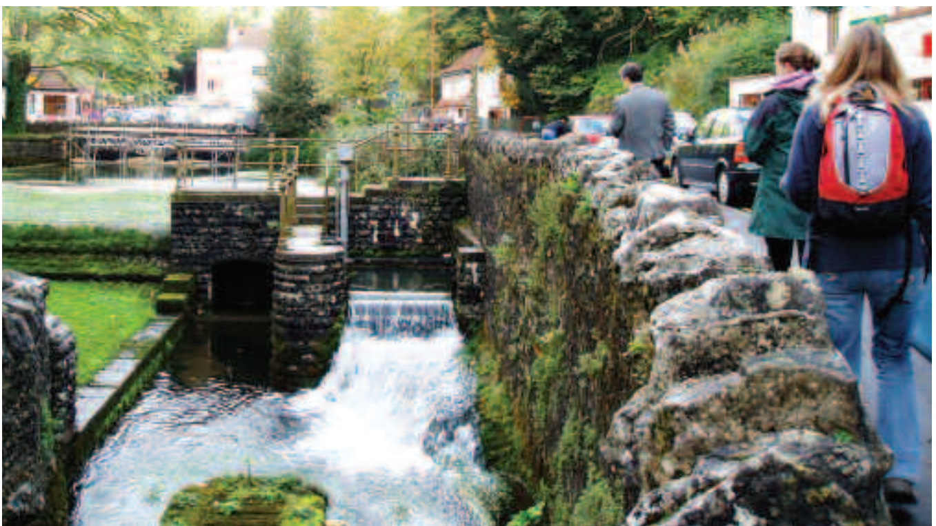
Compensation Weir at Lower Cox Mills Pond, Cheddar
