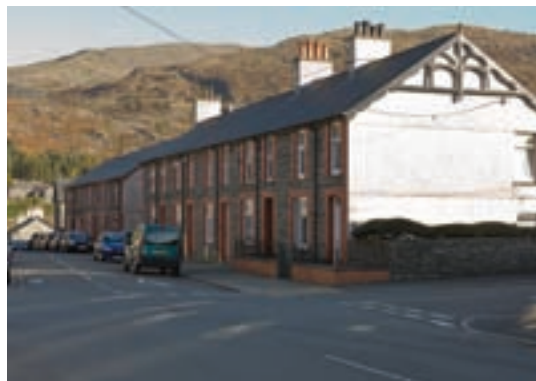
The use of brick dressings distinguishes housing on Wynne Road (Crown Copyright: RCAHMW).
