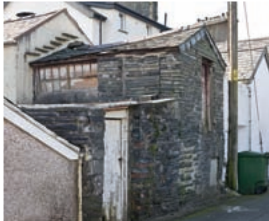
Slate as a walling material is rare in the town, but was sometimes used for outbuildings (far left) and ancillary structures (left) (Crown Copyright: RCAHMW).
