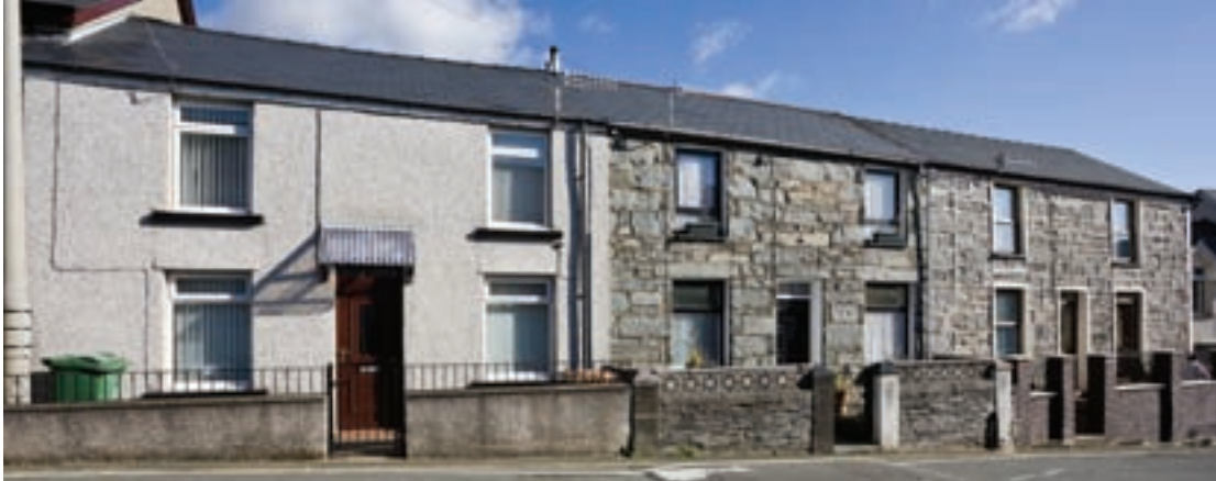
Missing chimneys, and modern render and window detail have eroded the original character of this terrace (Crown Copyright: RCAHMW).
