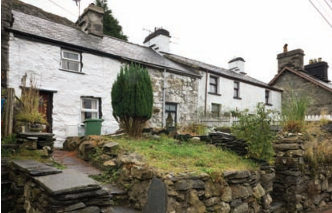
Limewash and rough stonework boundary walls (Crown Copyright: RCAHMW).
