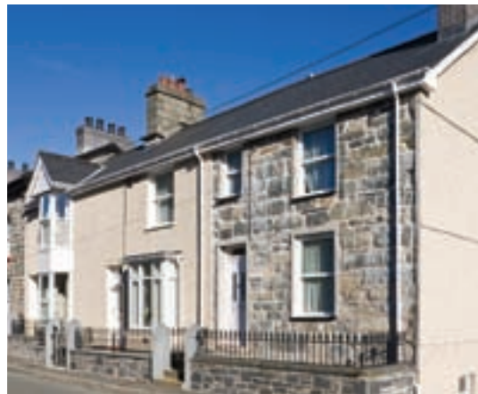
The uniformity of 1870s housing development is eroded by modern render (Crown Copyright: RCAHMW).
