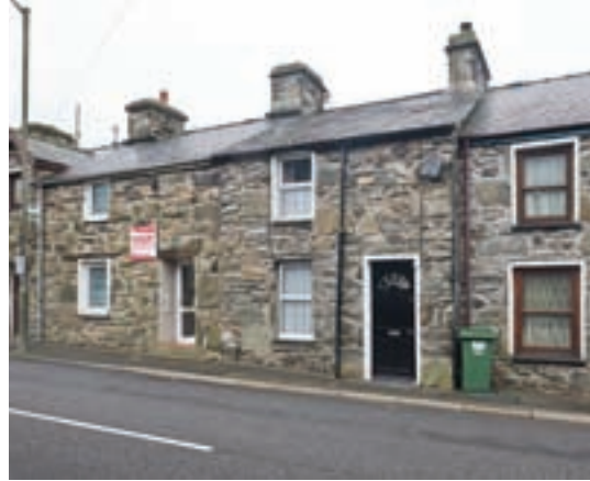
Urban housing along the main road whose line was completed in 1825. Differences in the stonework betray the fact that many terraces were the work of more than one builder (Crown Copyright: RCAHMW).
