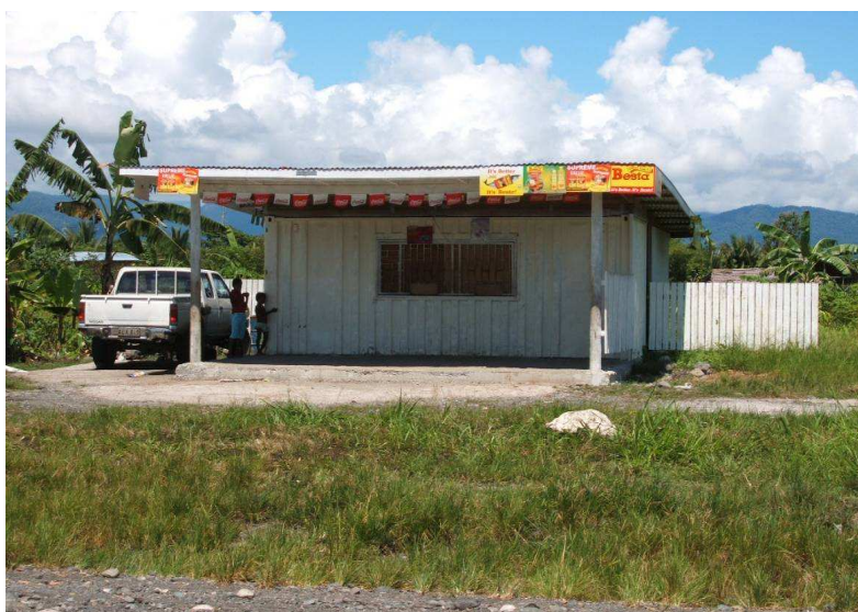
Figure 5: A shop situated on Portion 351 on the main Malahang road
