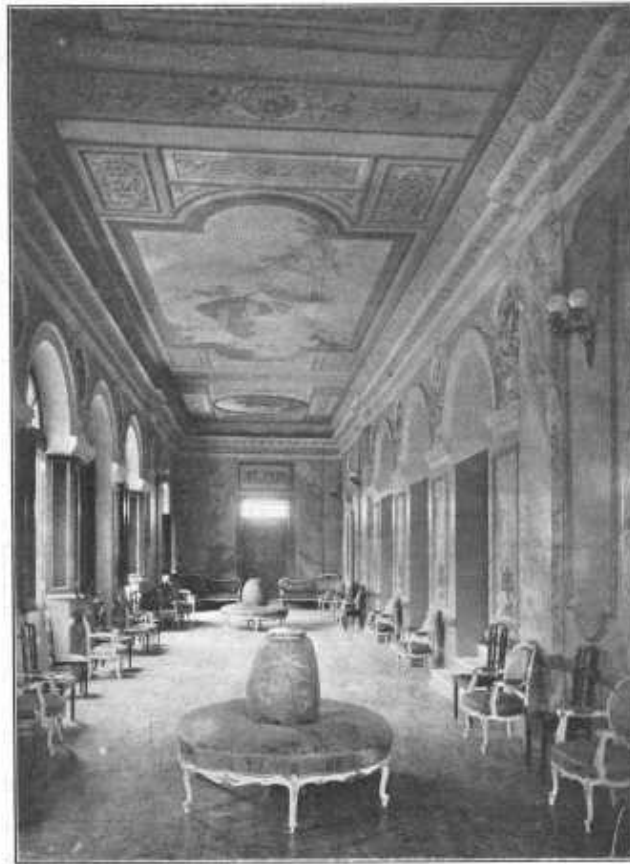
Foyer del Teatro Nacional National Theatre—Foyer
