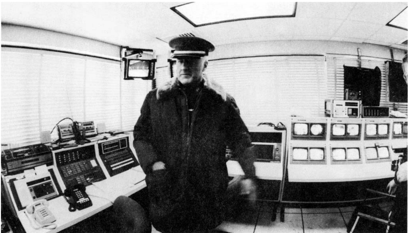
Closed circuit television system and other modern communications systems at the Olympic Village
