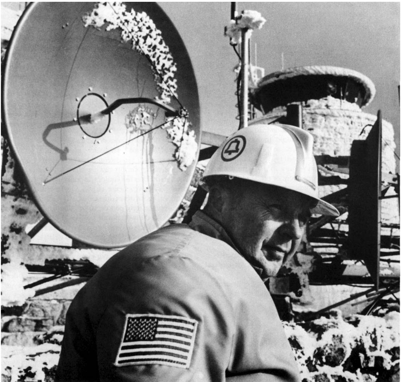
New York Telephone Co. supervising engineer for radio and TV stands at Whiteface summit, amid microwave system that beamed 1980 Winter Olympics around the world
