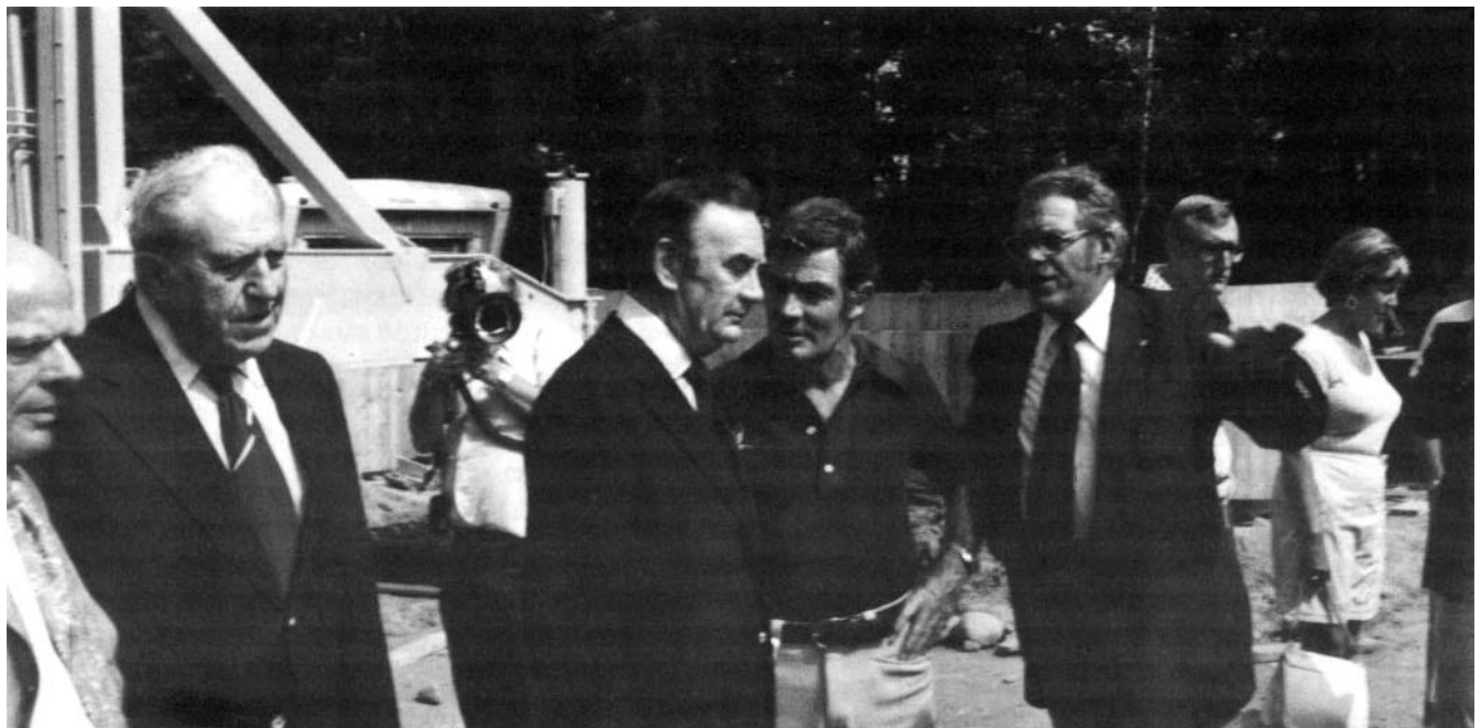
LPOOC officials tour construction sites with New York State Governor Hugh Carey
