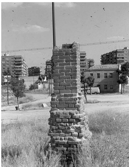
Figure 8. Breather. Alto Abroñigal qanat
