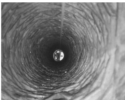
Figure 6. Breathing well. Fuente del Berro qanat
