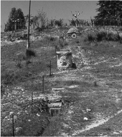
Figure 10. Course of the Rey qanat indicated by breathing wells
