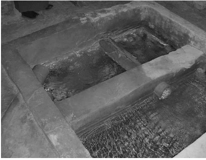
Figure 17. Main drain. Ocaña qanat
