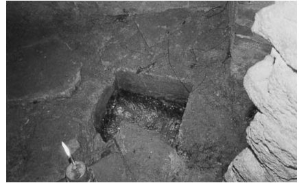
Figure 11. Registry drain. Fuente del Berro
