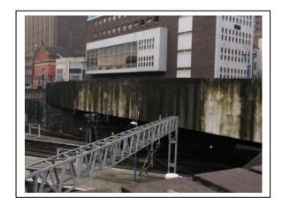
Pinfold Street/ Navigation Street/ Hill Street – currently a mix of blue and white to the internal surface of walls 9 and 10 (internal face of wall 9 shown in the photograph below), with wall 8 a brown engineering brick. It is proposed to re-paint all existing painted surfaces light grey and retain the brown-faced engineering brick as it is.
