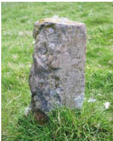
A marker stone on the line of the Bonaly to Edinburgh water pipeline at Dreghorn. Probably erected in the late 18th or early 19th century, this stone has been damaged by gunfire from the adjacent rifle-range. DP006704
