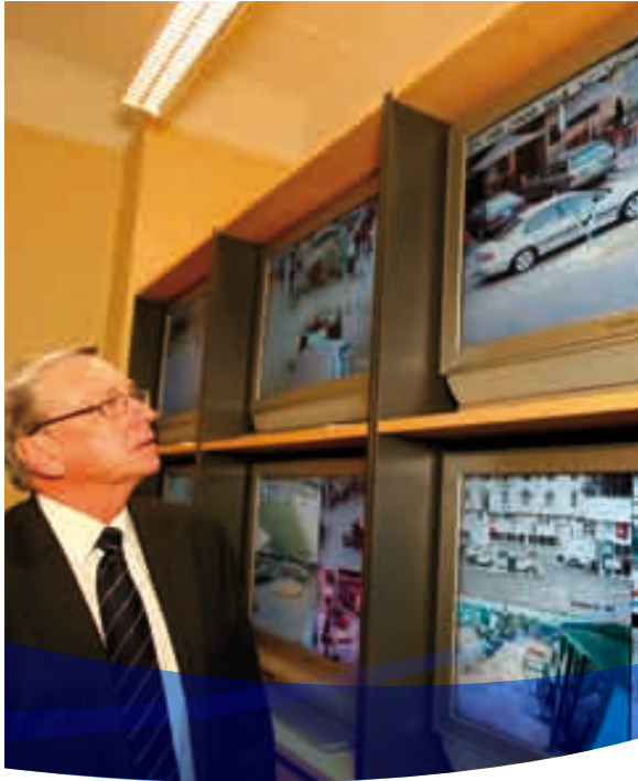
Minister Jim Cox MP in the CCTV viewing facility, Hobart
