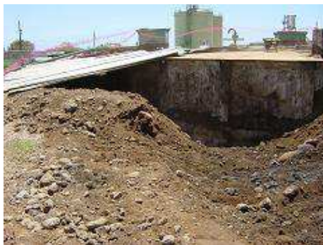
▲ Digging operations round the SEA2 tank (Photo DR)
