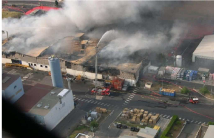
Spread of the fire to several buildings
