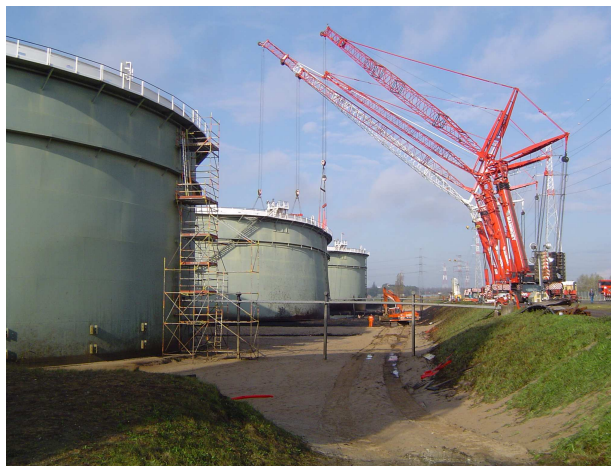
Figure 4: Major cranes stabilising tank D2
