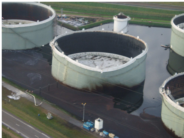
Figure 1 shows a picture of the situation in the bund the morning after the major accident happened.
