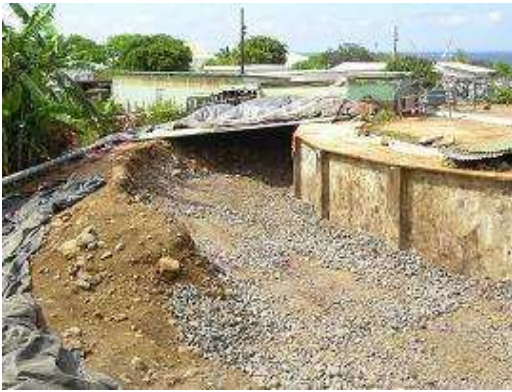
▲ Backfill around tank SEA2 (photo DR)
