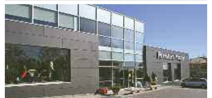
Ferreteria Maspor S.A. / 93 843 00 03
