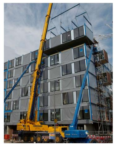
Modern Methods of Construction (MMC) offer significant potential to minimise construction waste. This report identifies the current use of MMC, the potential for further uptake and the waste minimisation potential.
