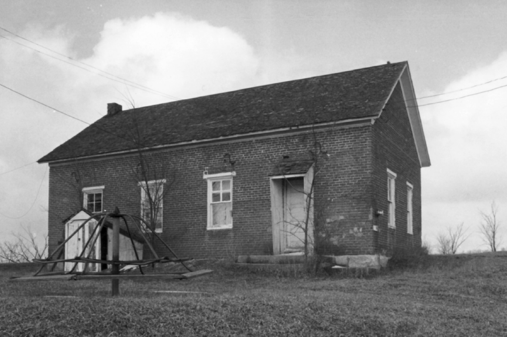
Photo 1 of 3. General view of main entrance (south) façade looking north-northwest. Photo by D. Murphy, 1976, NSHS (7602/2:36A)
