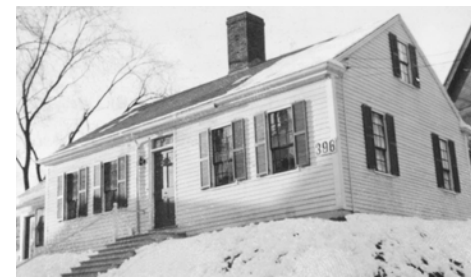
Smart-Daggett House Oldest House in Bangor
