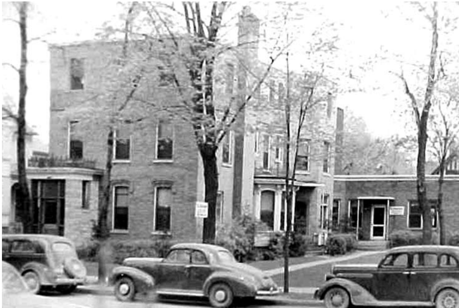
Photo C: A third floor and a new brick front façade made the old house look newer.
