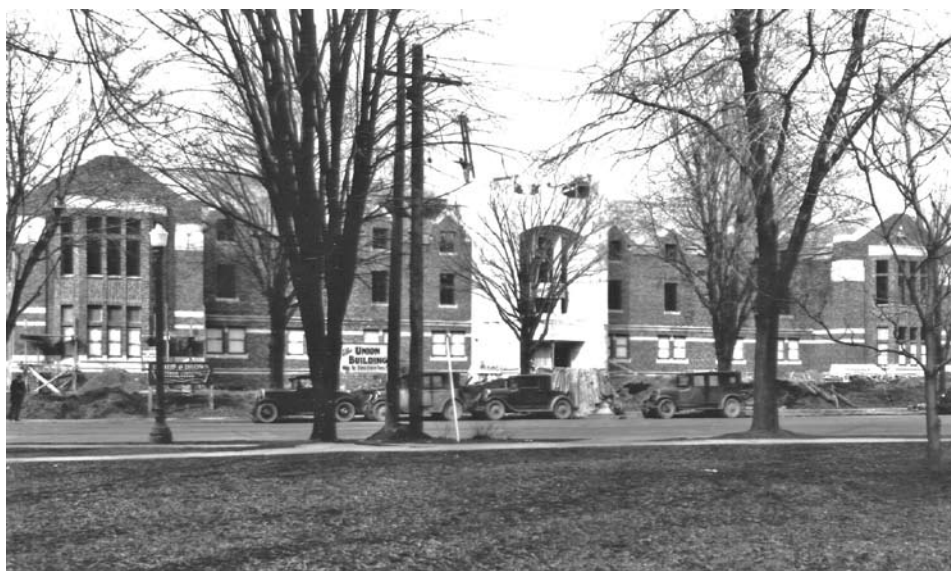
Construction of McKenny Hall, C. 1931.
