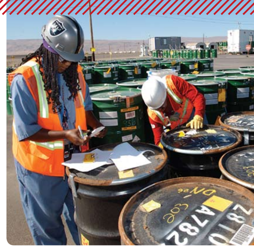
Environmental workers retrieve 55-gallon drums of radioactive waste from a burial site at Hanford's central plateau in 2005. (Photo: U.S. Department of Energy)
