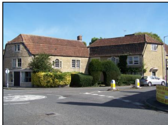
Pantiled mansard roofs on nos.1 & 3 Warminster Road
