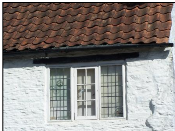
Casement with timber central opening flanked by leaded lights at no.7 Warminster Road
