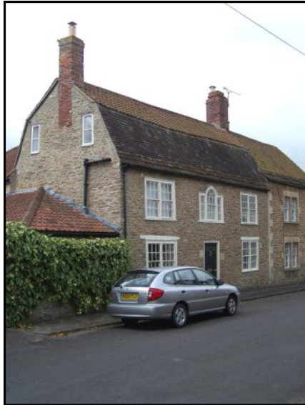
Venetian window and sashes at no.66 Goose Street
