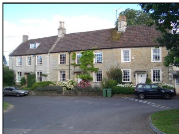
Typical sash windows at nos.19-23 Castle Corner
