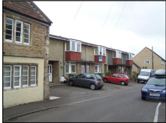
Modern development on Goose Street
