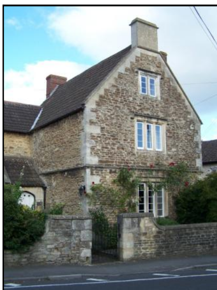
17th-century mullioned and labelled windows at The Hawthorns, no. 20 Bath Road
