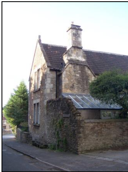
Coped gable and massive chimney stack, The Old Church House, Church Hill
