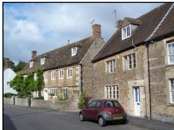
Stone tiles and pantiles, hipped and gabled dormers on Goose Street
