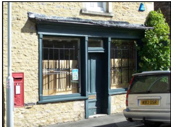
Shopfront, Warminster Road
