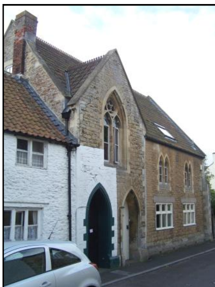
Nos.4 & 6 Goose Street, the former Enderby Hall
