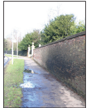
St John's boundary wall
