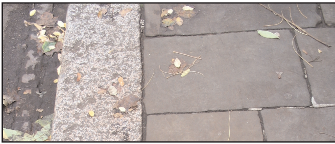
Paving on Trinity Lane
