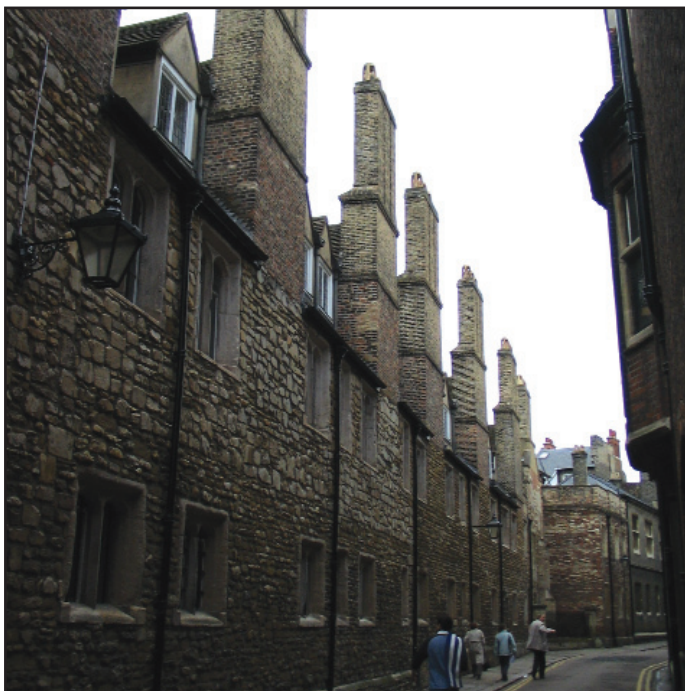
Trinity Lane chimneys
