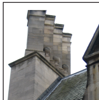
Trinity Lane chimneys
