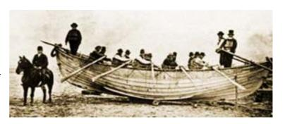
The Zetland is a clinker-built boat of oak frame and larch planking 9.15 (30 ft) long with a 3.1m (10ft) beam. She Originally had a thick cork band (fender) running around the top of the boat but this was later replaced with extra internal buoyancy tanks.
