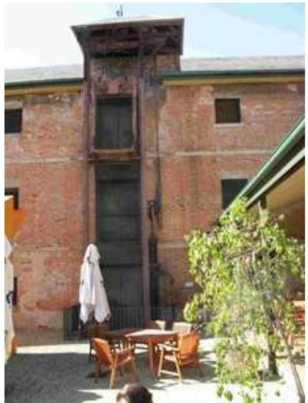
Figure 13. Goods Lift, Hobart Bond Store building (Photo – B Cole)
