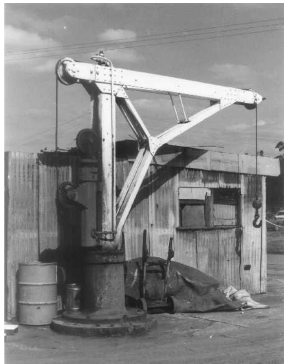
Figure 12. Hydraulic Crane Newport Railway Workshops. (Photo – C & M Doring)
