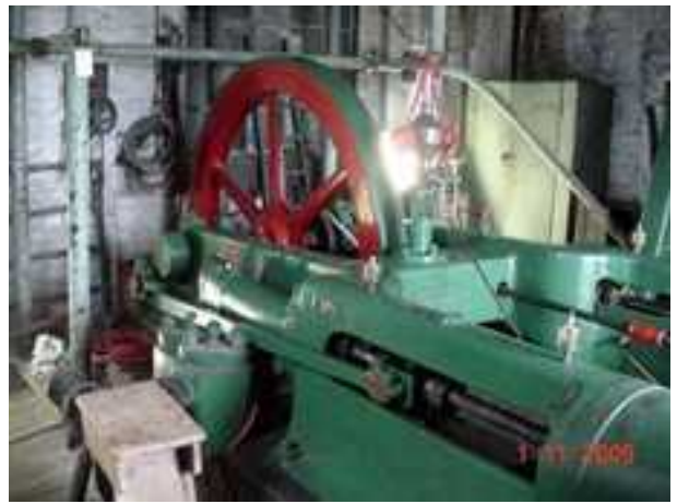
Figure 4. Fielding & Platt HP Pump, Chullora.
