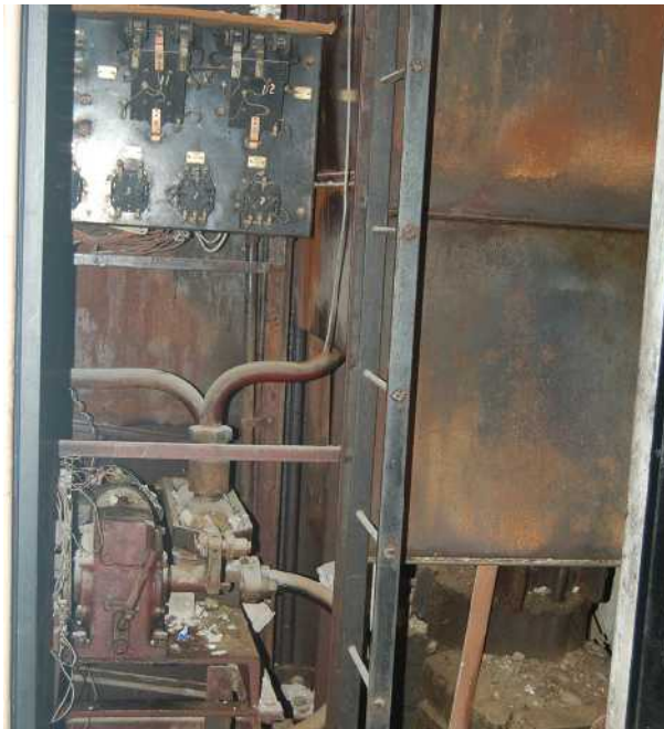
Figure 14. Electric Control for Bullion Lift.
