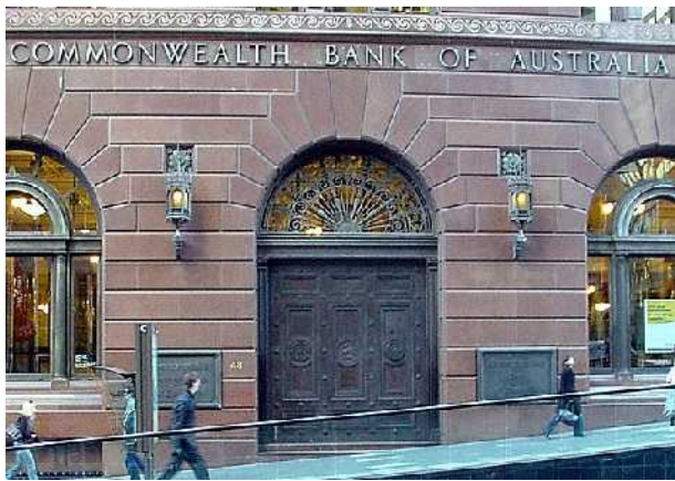
Figure 22. Hydraulically operated Bank Doors, Sydney.
