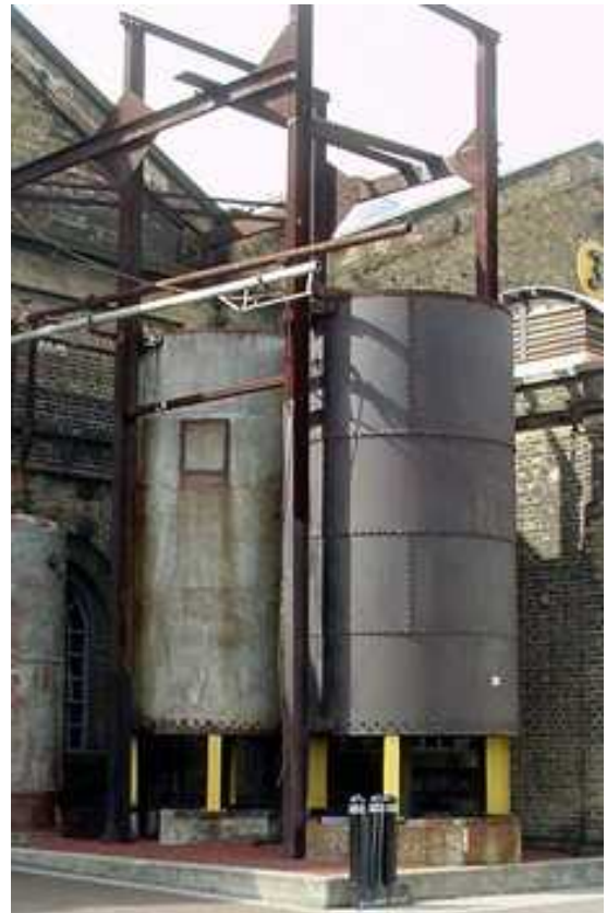
Figure 7. Accumulators, Eveleigh, Sydney.
