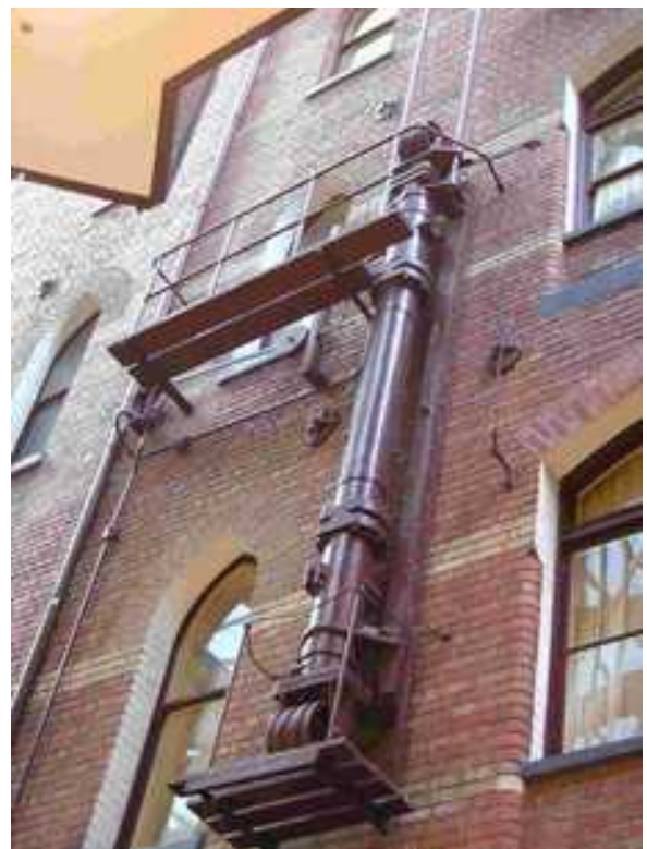
Figure 10. Rialto Building Hoist (Whip), Melbourne.
