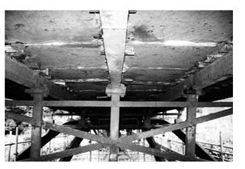
*Figure 18: Typical inverted 'T' beam bearer, supported by the spandrel frames transverse tie beams.*
