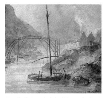
Figure 11: The Martin sketch identified two standing derricks with a cross bar: in essence forming a simple crane. (Skandia Insurance Company Ltd, Stockholm, Sweden, photographed by Ake Cyrus).
