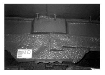
Figure 5: The rear view of the crown which locks all the major components together, thus guarding against vertical and lateral movement. These components clearly show the up-cast and down-cast faces of the ironwork (Ironbridge Archaeology Archive – F13/8).
