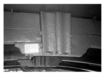
Figure 6: A front view of the crown joint showing the crown bearer and upper ribs A and B (Ironbridge Archaeology Archive -F9/10).
