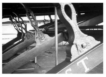
*Figure10: A view across the five frames of the bridge, showing at least two of the differing radials.*
