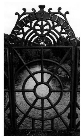
Figure 15: The centre panel of the bridge parapet with initials of John Onions, who supplied the ironwork for the 1818 bridge.
