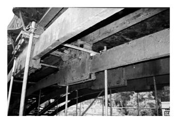
Figure 17: Fishplates connecting the centre span ribs.
