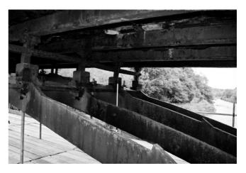
Figure 16: Ribs 2, 3 and 4 showing the redundant lugs of 1800.
