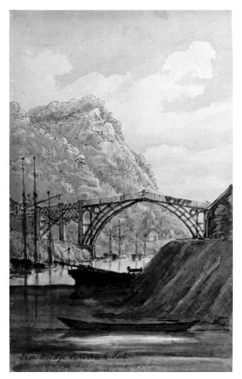
*Figure 4: 1804–21 Pencil sketch showing the first large-scale alteration of the bridge with wooden trellis arches in the South Abutment. (Ironbridge Gorge Museum Trust – CBD 1978.225).*
